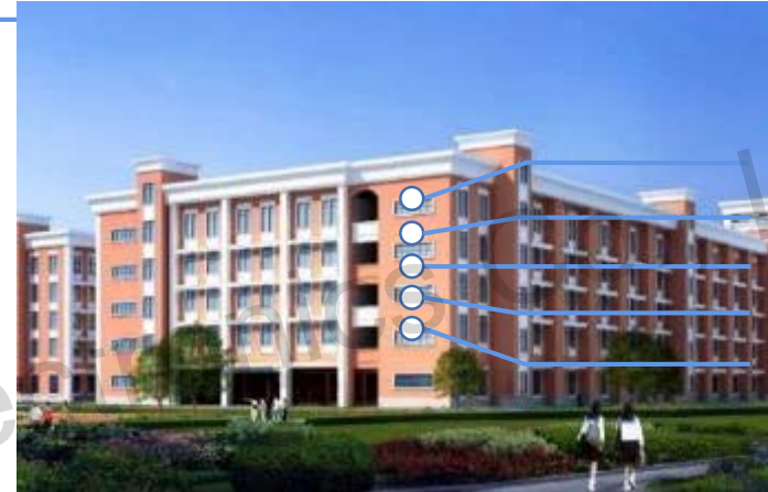
Middle school building
