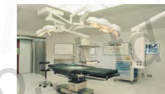
Duty room, control room and operating room
